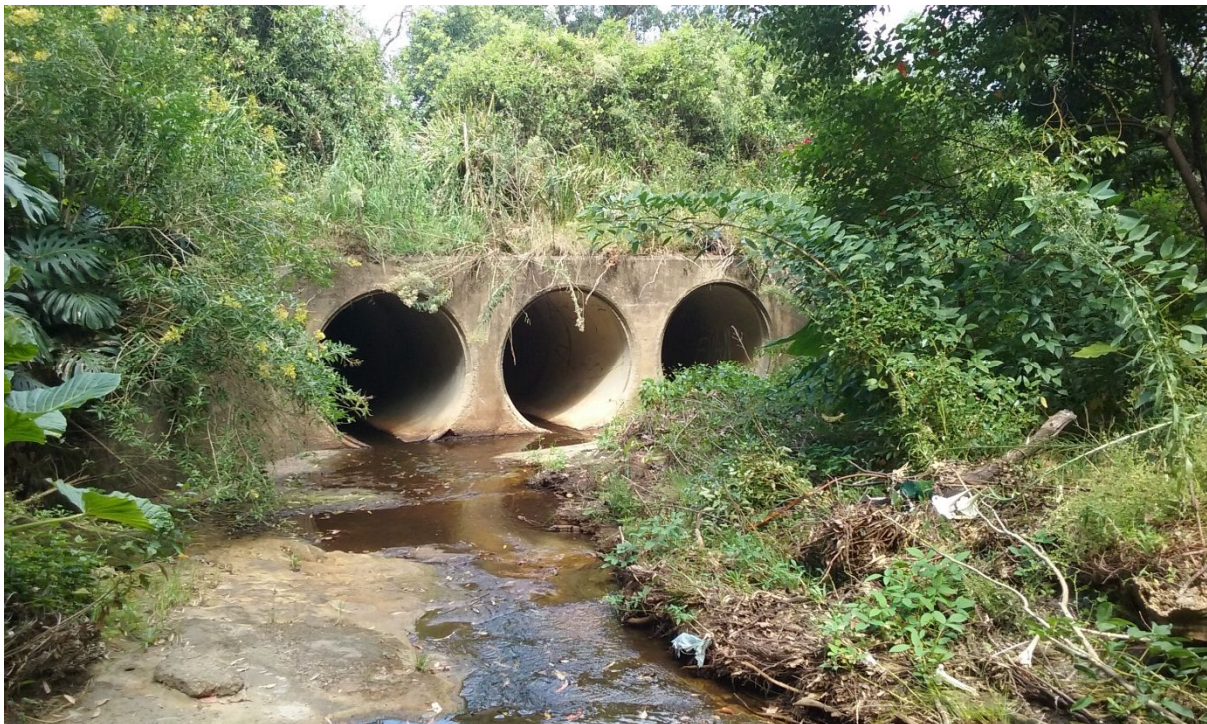
Figure 7 Culvert on Mullet Creek, under Powderworks Road
